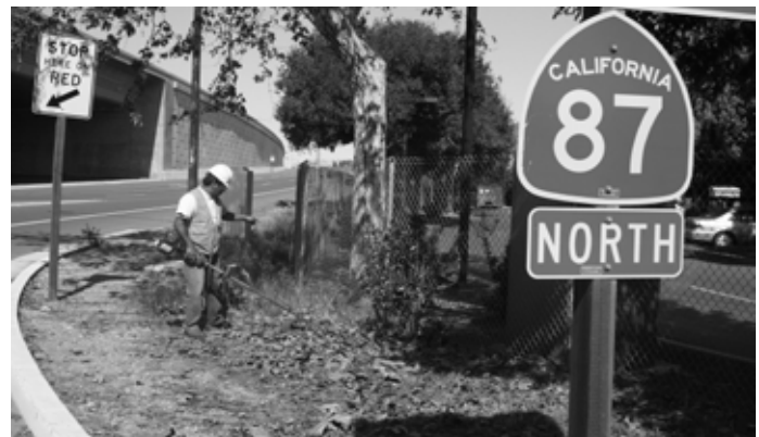
Removing weeds at Hwy 87 on ramp.
